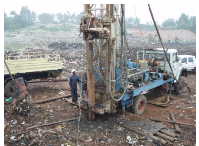
Drilling for methane gas monitoring well in 2010 as a German project
