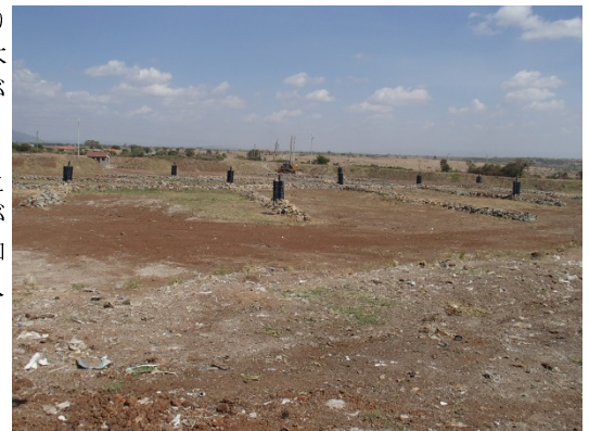
Pilot landfill in Thika – main body is well maintained in the same way as last year and greening of the embankment is expanded
