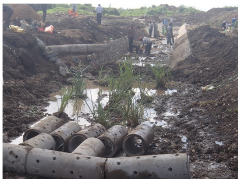
Biotores were also set up with locally available water grasses (for biological decomposition of leachate's organic matters)
