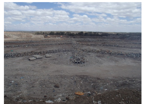
Completion of installation of perforated pipes / 完了した穴開き管の敷設
