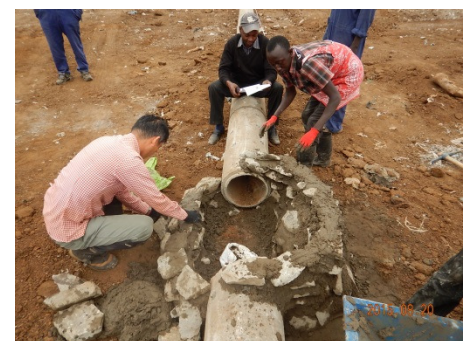
Application of mortar to stonework / 石積みにモルタルを施工
