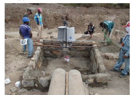
Leachate treatment facility (under construction) / 浸出水浄化施設 (建設中)
